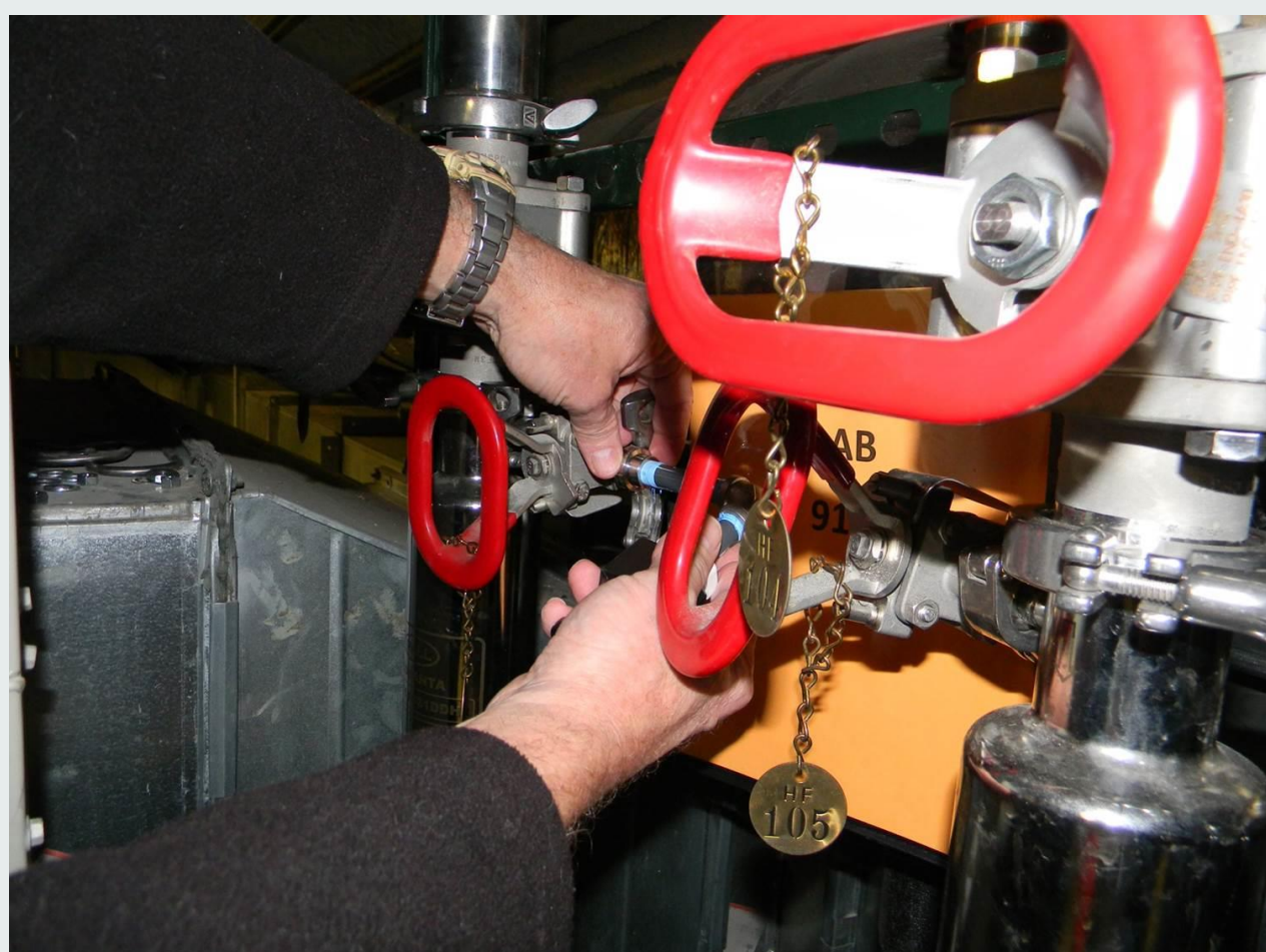
Connecting adapter to test port
