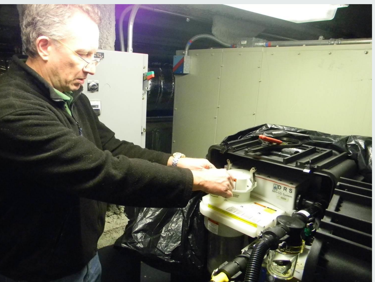
Adding CD Generation Chemicals and Neutralizer Tablets to the MCS
