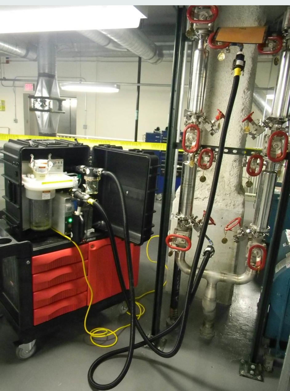
MCS connected to one side of pall filter array
