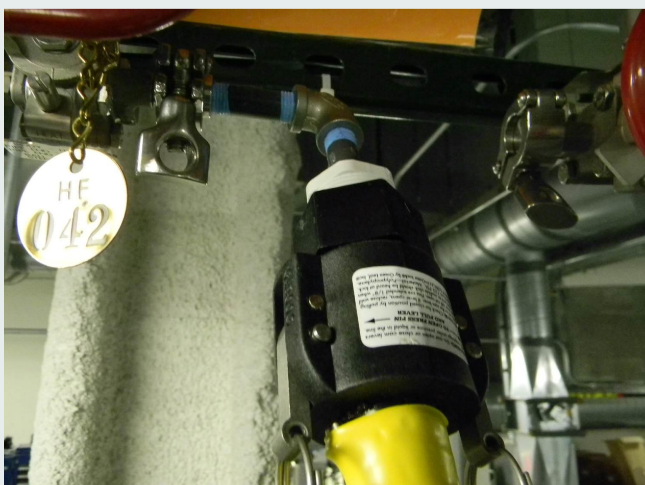
CD Supply hosing connected to upper test port
